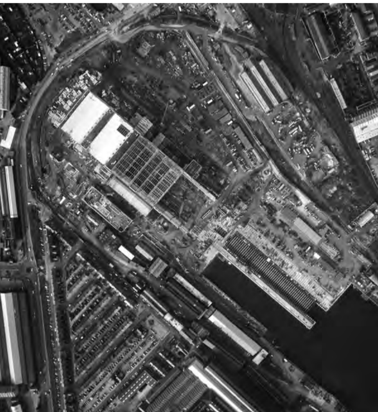
● Above, the view from the air of the Devonshire Dock Hall at Barrow in May 1985; Below, the Royal Naval College at Greenwich, London, in 1946
