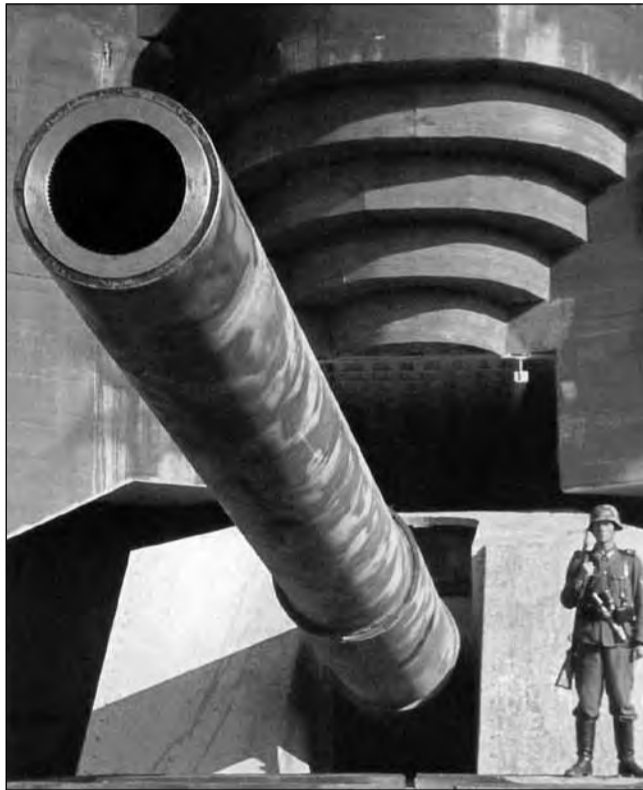
● One of the four 152mm naval guns at the Longues-sur-Mer battery between Gold and Omaha beaches. Part of Hitler's Atlantic Wall, the battery was completed less than two months before D-Day, and was out of action by 7pm on June 6 1944
