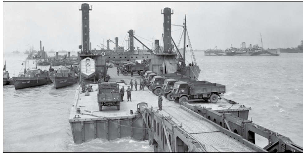
● Lorries are loaded at a pierhead in Mulberry B at Arromanches during June 1944
