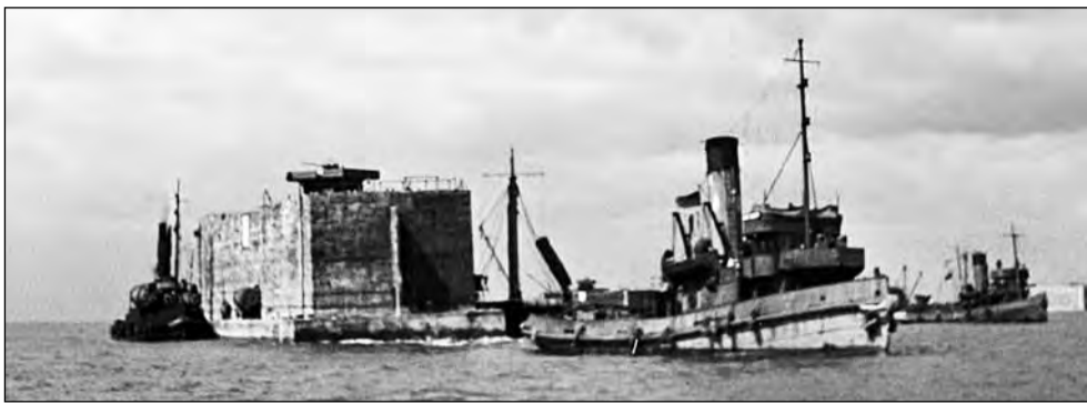
● A Phoenix caisson, with gun tower on top, under tow, possibly at Dungeness or Pagham
