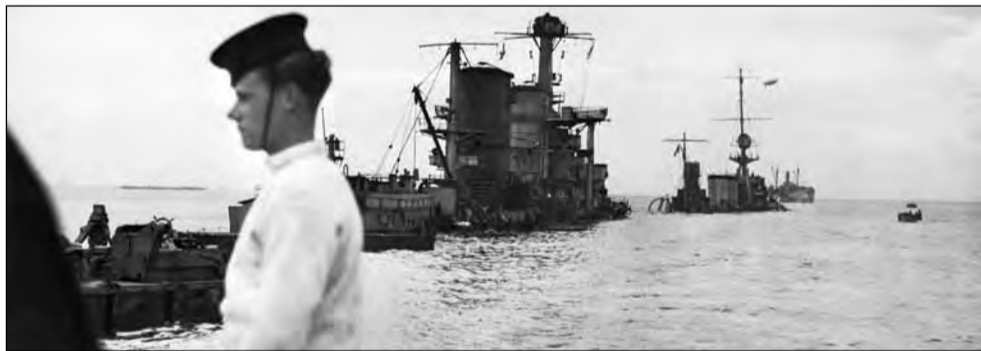
● The Gooseberry breakwater off Sword beach, which included the old cruiser HMS Durban (pictured) as well as French battleship Courbet (Picture: © IWM (A 24054))
