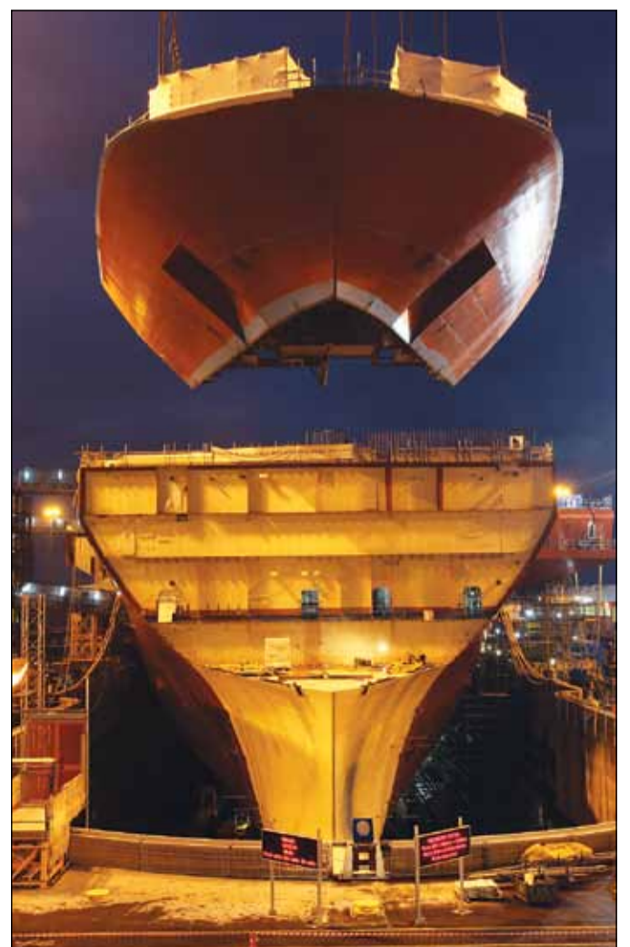
● Today's giant piece of the Queen Elizabeth jigsaw is sponsored by a well-known mobile phone manufacturer... A Portsmouth dockyard worker takes a shot of the forward island before it leaves the Solent by barge and (below) the middle bow section is lowered into place on a chilly night in Rosyth
