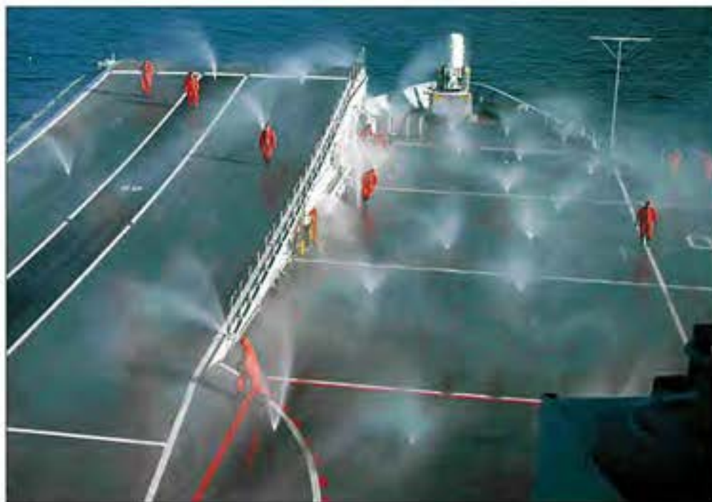
I guess the hosepipe ban is over... Ark's crew check her flight deck sprinkler system during a 'pre-wet' test
