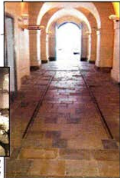
● Right: The rail tracks inside the central arches that were used to transfer patients and kit around the hospital
