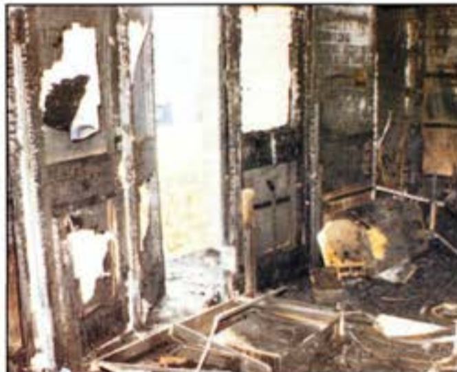
● Gutted: the charred remains of TS Obdurate, Warrington
