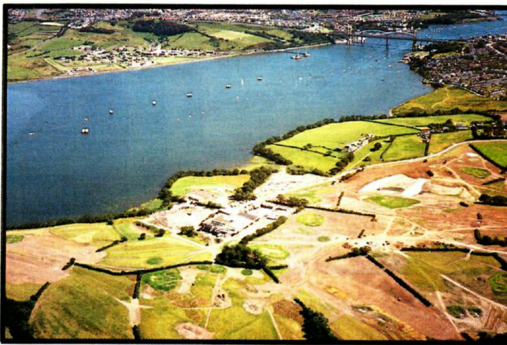
● Aerial view of the 180-acre site, including the Cornish cottage complex under construction, and the 18-hole, par 72 golf course, with Devonport naval base and the Tamar Bridge, top right.
