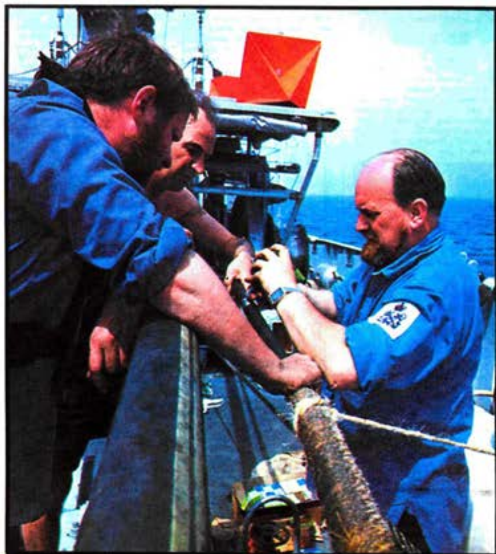
Clyde Division men repair loop wires on board HMS Crofton.
