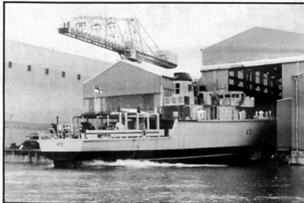
Gathering pace down the slipway, HMS Dulverton leaves her covered berth at Southampton.
