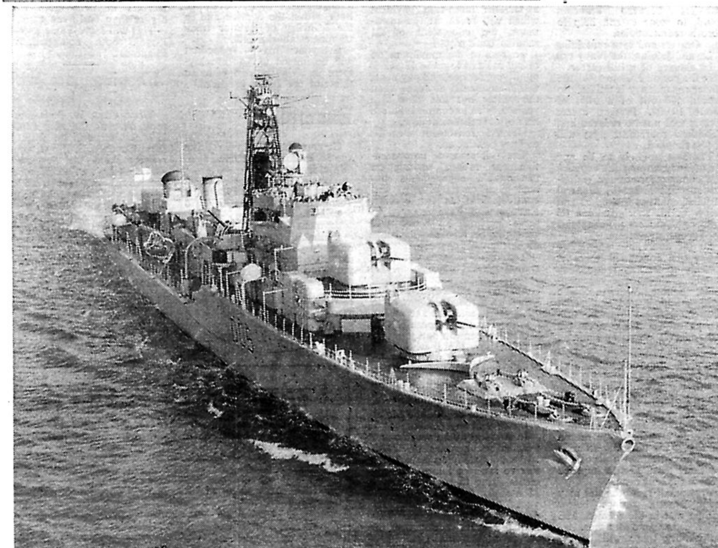
Two Daring class destroyers are open to visitors at Portsmouth—the Defender and Decoy—and H.M.S. Delight will be at Plymouth but not open to visitors. H.M.S. Daring (below) displaces 3,600 tons (full load) and was built between September, 1945, and March, 1952. She was modernised 1963/64 when the torpedo tubes were removed.
