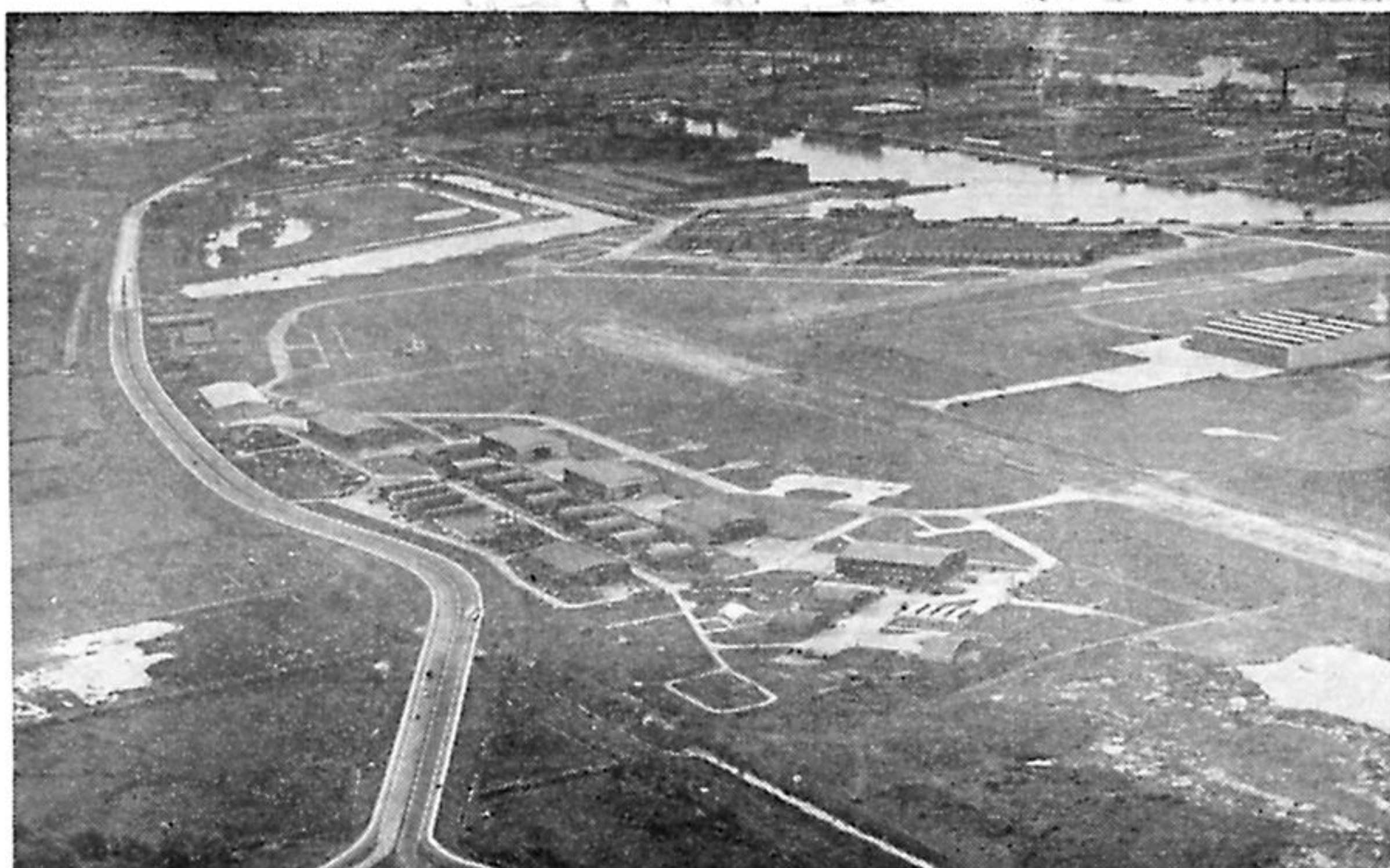
R.N. Aircraft Yard, Belfast. The hangars and workshops are grouped in the foreground close to the new Sydenham by-pass road. The shipbuilding yard of Harland and Wolff and Belfast docks can be seen in the top right-hand corner. (Photo.—By courtesy of "Belfast Telegraph")
