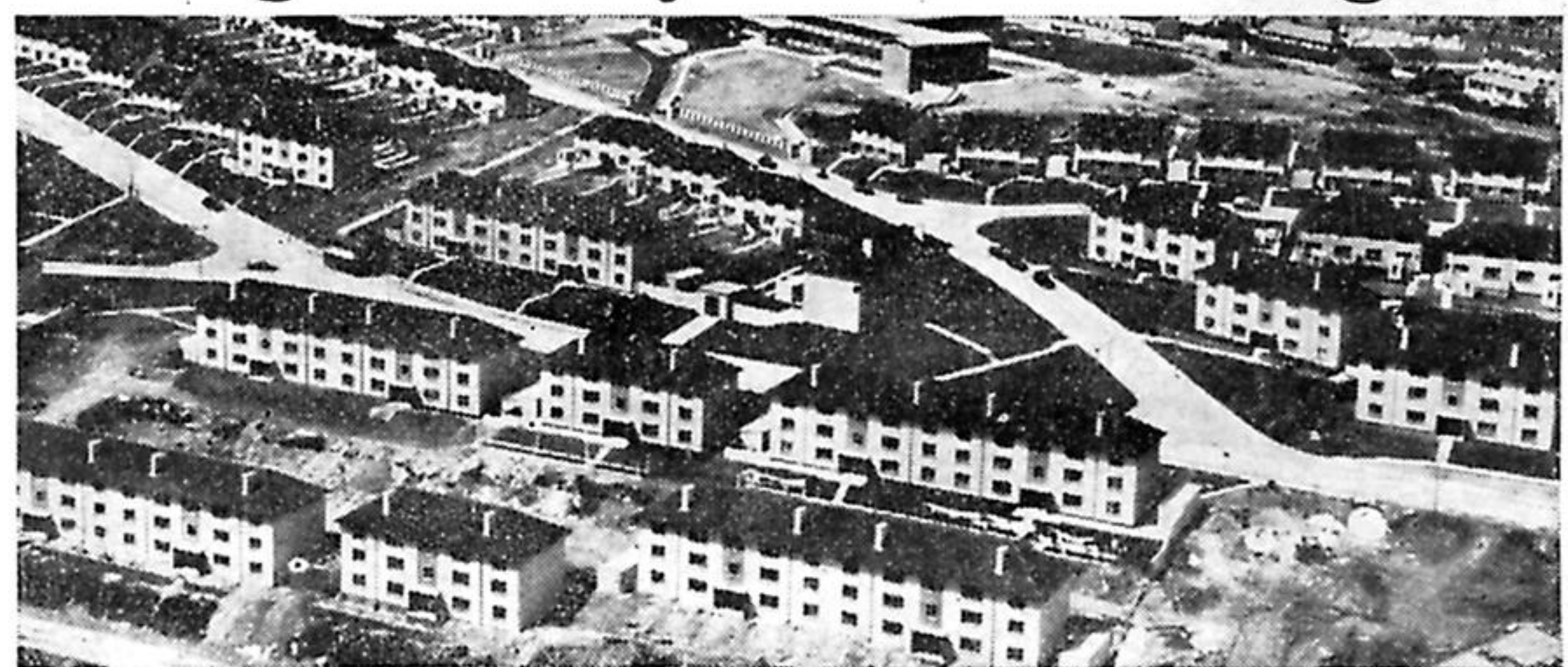
Blocks of flats on well-laid-out estates have gone a long way to reducing the waiting list for naval personnel at Devonport
