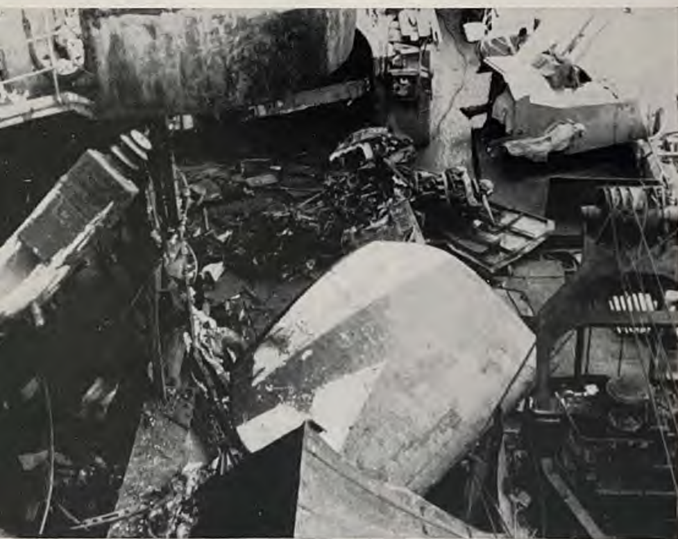
Damage on the aircraft deck (Hit No. 7).
