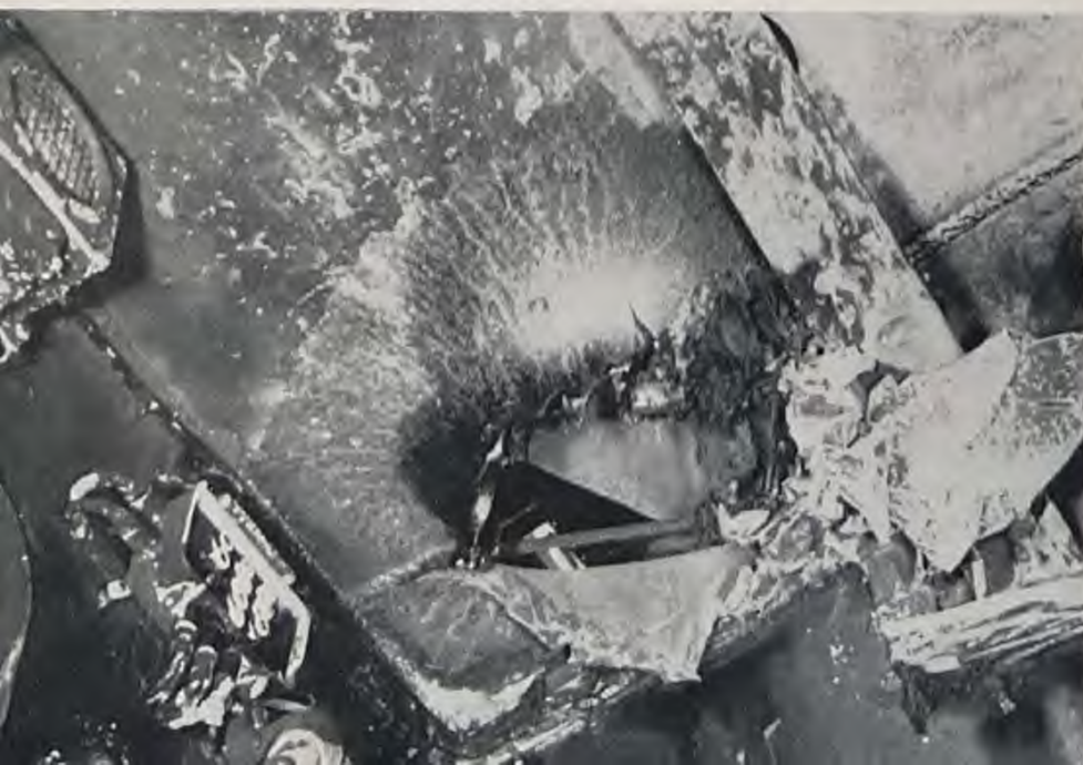
Bomb hole in upper deck (Hit No. 9).
