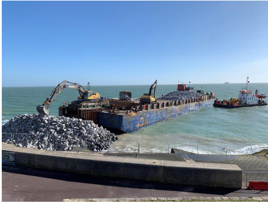
Delivery of rock armour to Southsea
